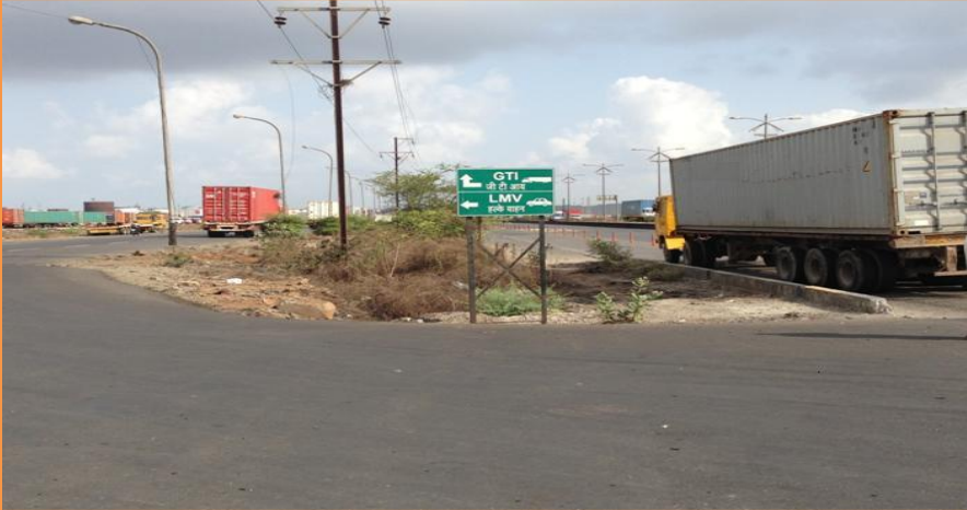
Dedicated approach road for APM Terminals Mumbai (GTI)
