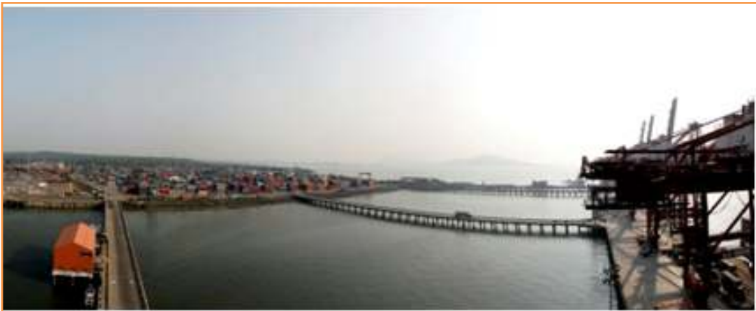
North-South-Central bridges connecting APM Terminals Mumbai yard to the wharf
